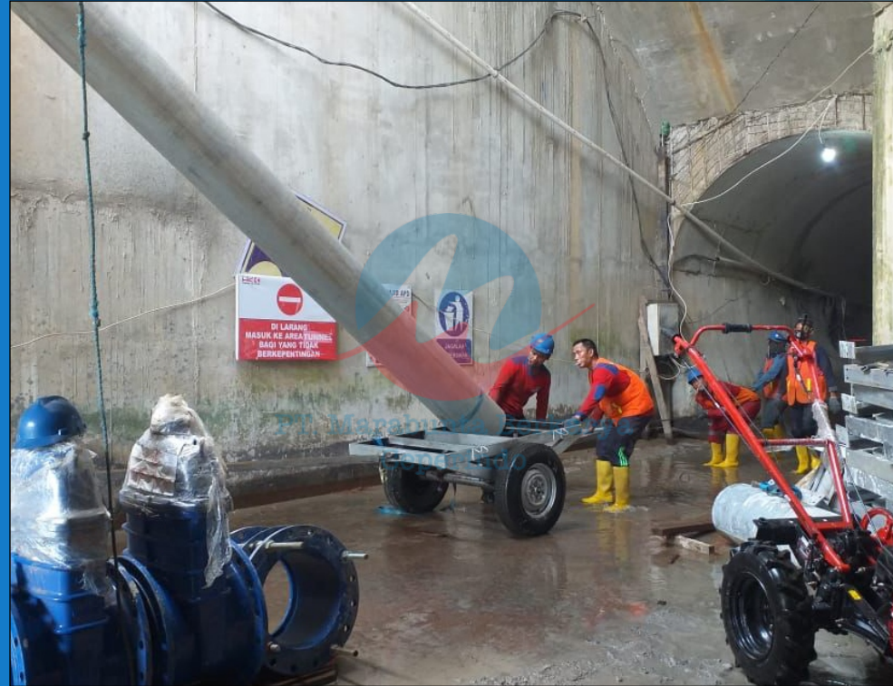
LOADING OUT PIPA HIDROMEKANIKAL
