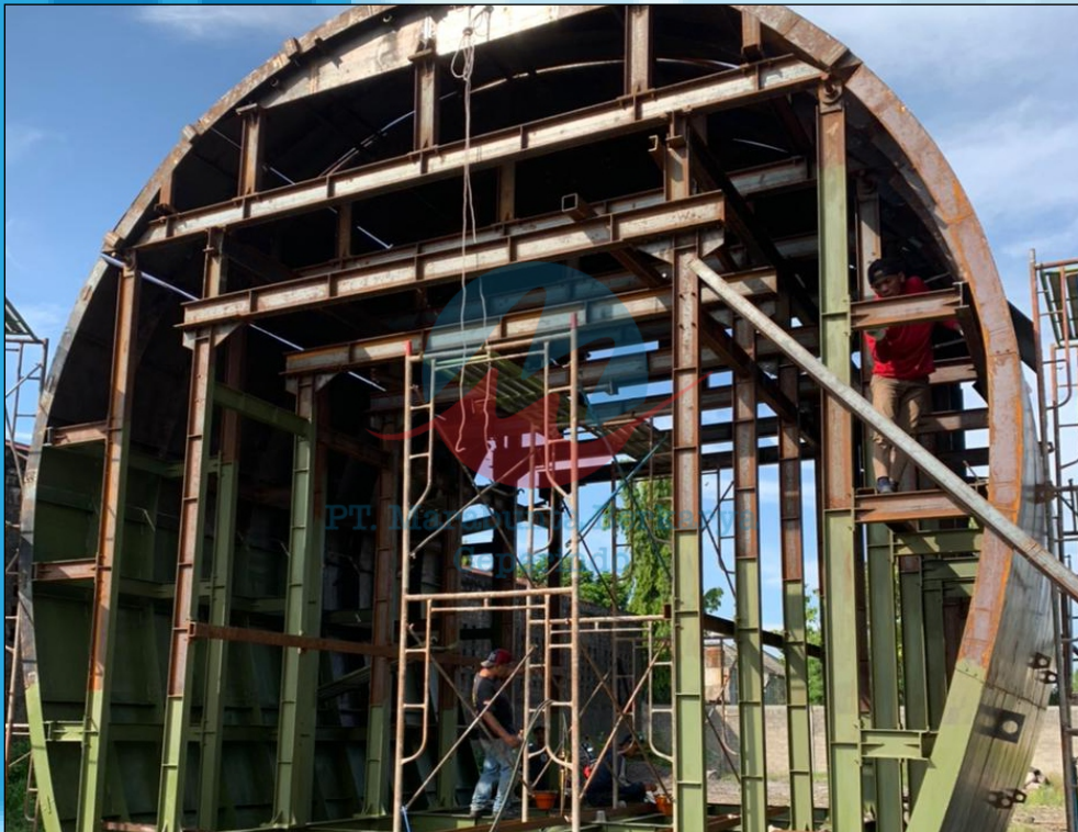
ASSEMBLY PART SLIDING FORM
