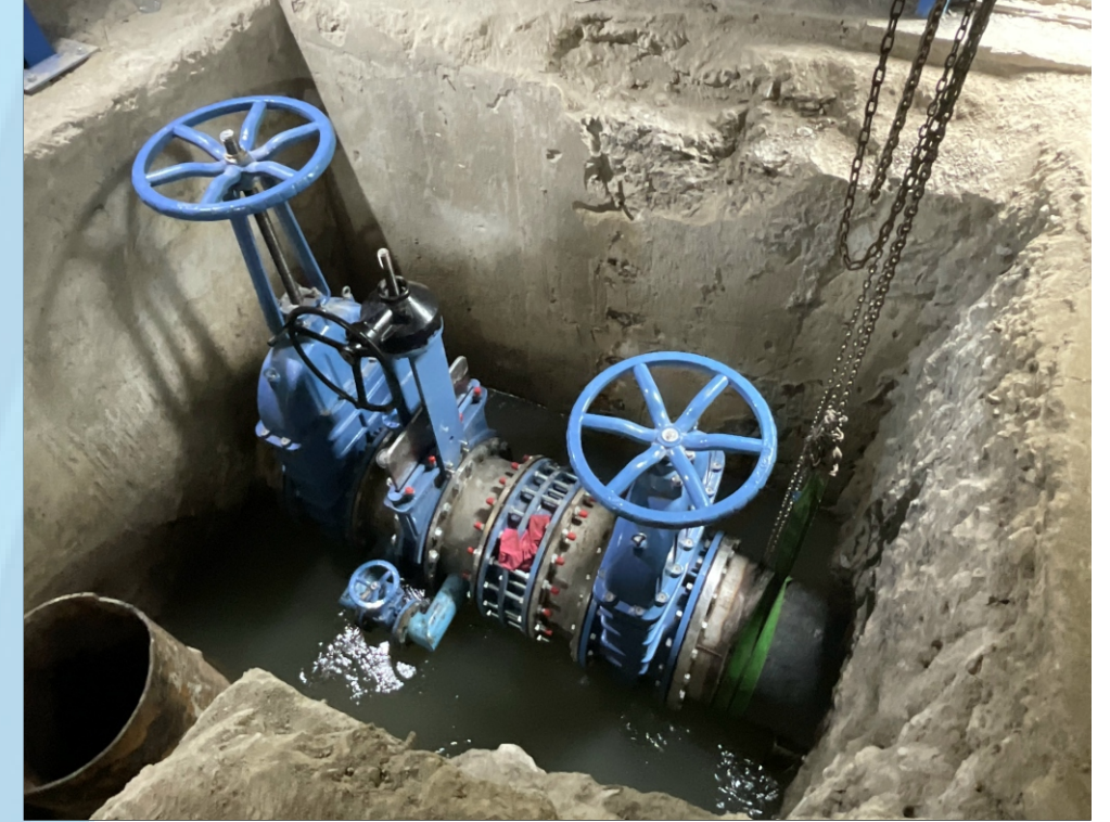
FINISH INSTALASI BONATED VALVE, KNIFE VALVE, GATE VALVE DAN DISMANTLING JOINT DN600 BENDUNGAN GONGGANG
