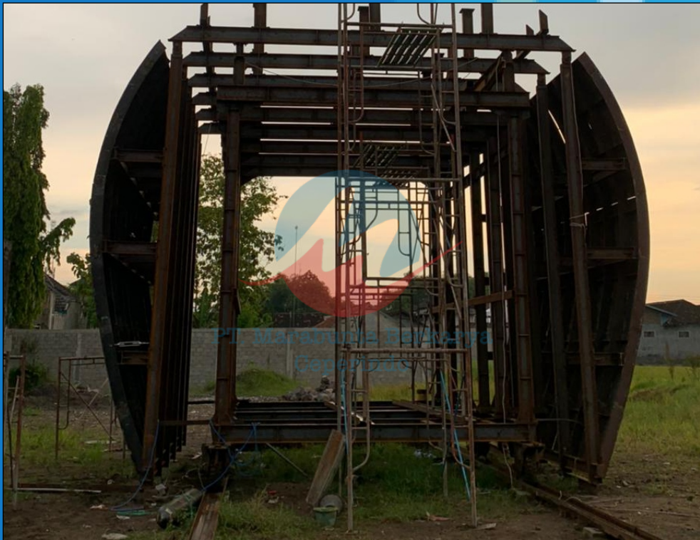
ASSEMBLY SIDE SLIDING FORM
