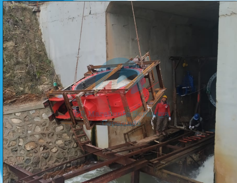
LOADING OUT BUTTERFLY VALVE DN1600 BENDUNGAN LADONGI
