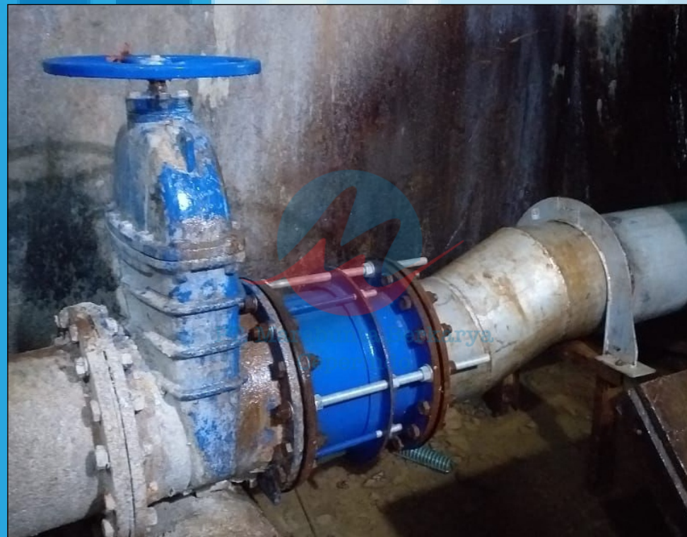
PEMASANGAN SADDLE SUPPORT
